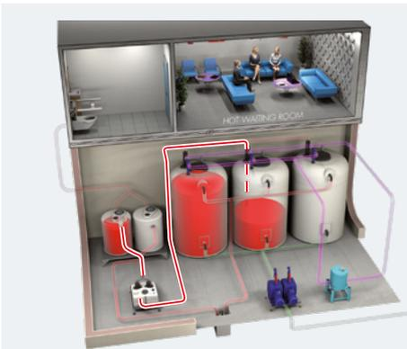
4) **Clarified water sorting at decay tanks:** this units allows collection and decay of radioactive liquid coming from the sorting unit.
