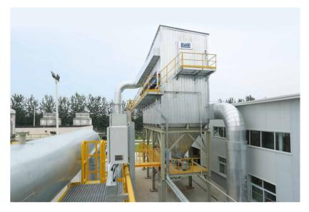
Catalytic candle filter for simultaneous reduction of pollutants.
