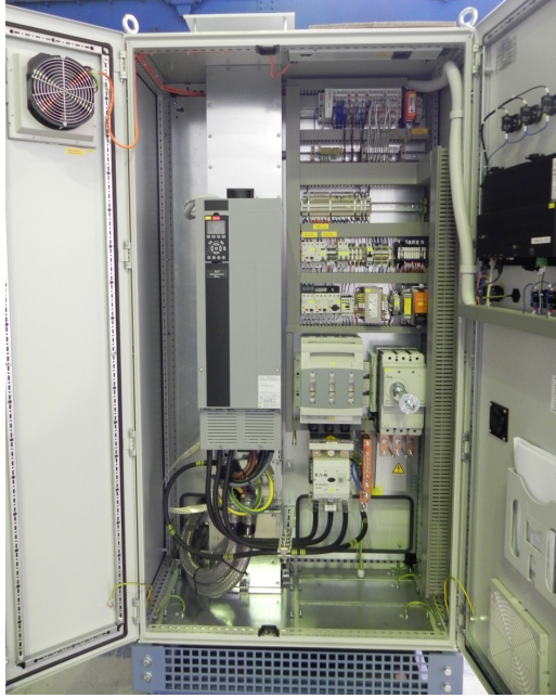
Fig.12: GEA Omni control cabinet interior view (frequency converter installed in control cabinet)
