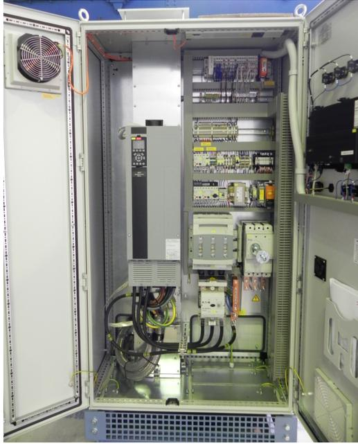
Fig.14: GEA Omni™ control cabinet interior view (frequency converter installed in the control cabinet)
